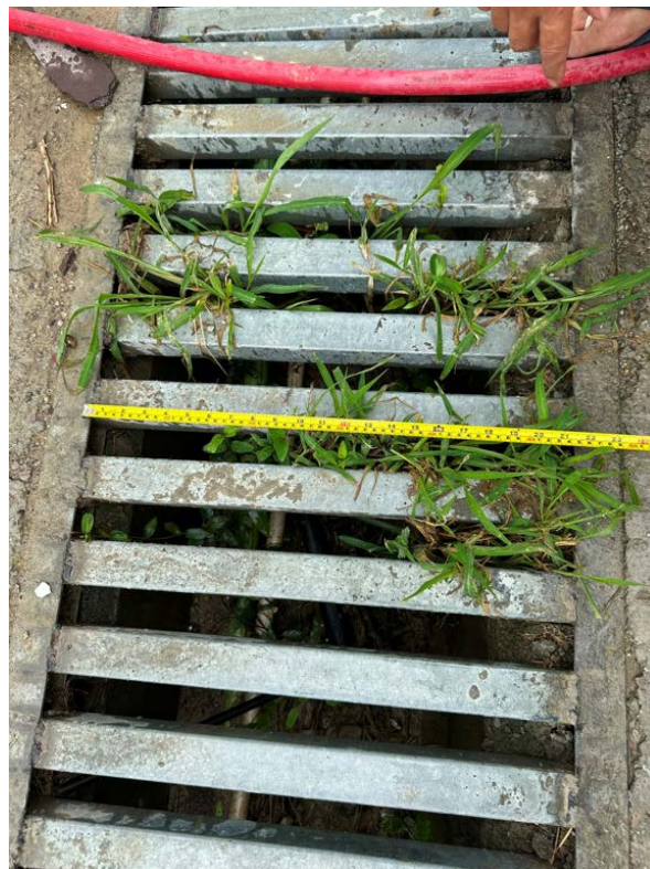
VIE 5: Existing 500UC on site
