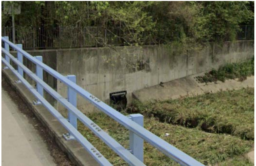
VIE 3: Existing 900mm dia. underground pipe
